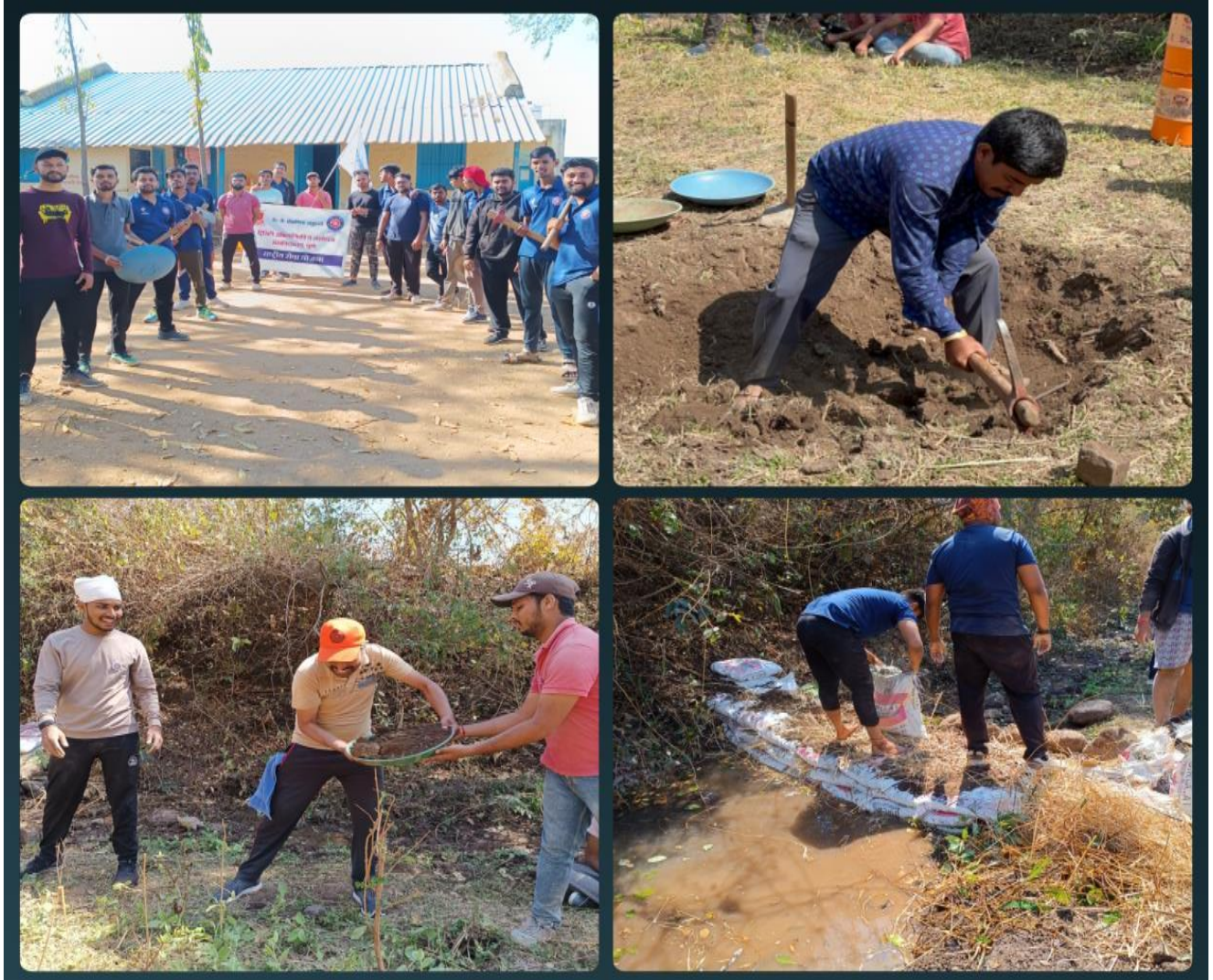
Building Check Dam
